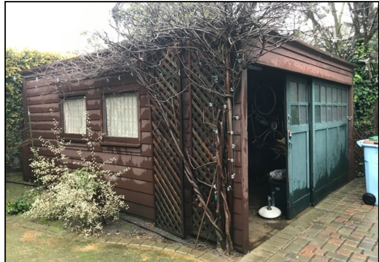
Garage before remodel.
