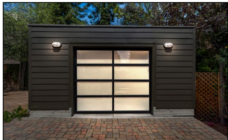
Exterior style of the garage mimics the main house to make it an extension of the home.
